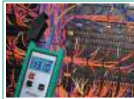
Fiber optic power test
