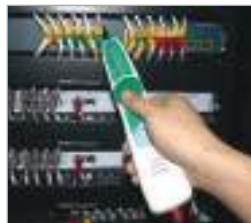
Copper cabling detecting
